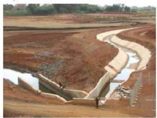
Figure 2.5: Koga Dam a) Koga Off-take towers b) Koga main irrigation channel and return flow to stream
