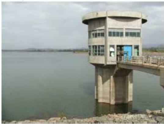
Figure 2.5: Koga Dam a) Koga Off-take towers b) Koga main irrigation channel and return flow to stream
