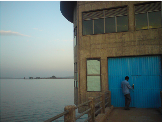
Professionals manage the infrastructure.
