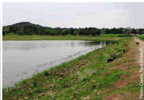
1b. Small dam/reservoir.
